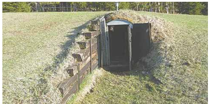
John Richards used a fiberglass septic tank to make an inexpensive cold storage cellar. He dug a hole in a sidehill near his house and buried tank.
