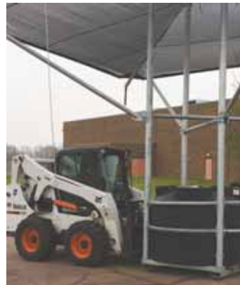
Shade is fitted with a 625-gal. water tank that serves as a base weight.
