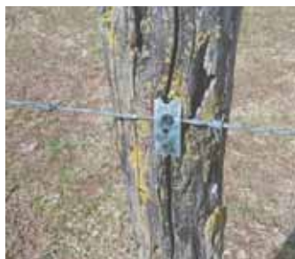
Perforated metal hanger straps are cut into 1-in. wide strips and then placed over wire. A cordless drill is used to drive screws through holes in straps.
