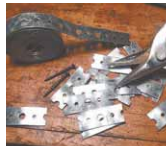
Perforated metal hanger straps are cut into 1-in. wide strips and then placed over wire. A cordless drill is used to drive screws through holes in straps.
