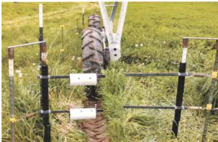
Electrified strap irons on one side of tower are fitted with two 4-in. dia. pvc pipes that ride over smaller pipes inside. Pipes turn freely to roll over pivot tire cleats without catching.
