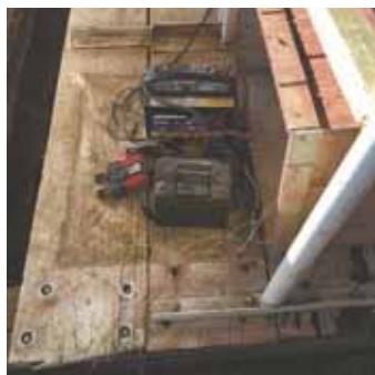
Portable solar-powered setup provides pond water to Cox's cattle. Four 40-watt solar panels are wired to a pair of 12-volt batteries located inside box on platform.
