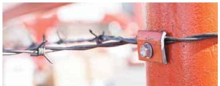
Clamp is curved slightly inward and has a small hole in the middle. Wire is inserted behind clamp, which is then screwed down tightly.
