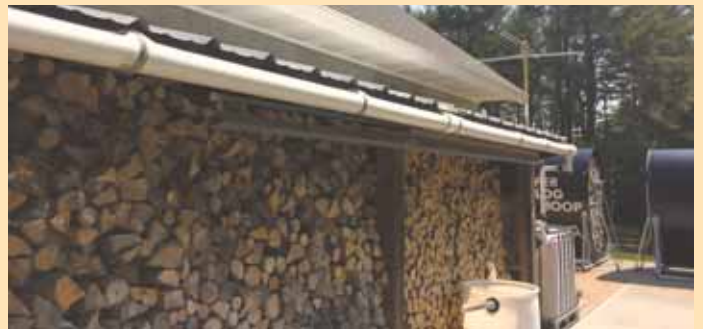
Smith cut notches into 4-in. pvc pipe and attached it to the eaves of his garage. Water flows off roof into a drop pipe that's plumbed to a pool filter, and then into tanks.
