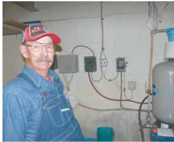
Howard Ewen uses tile lines laid around his farm buildings to capture drinking water. Tile is set in rock in a plastic-lined trench beneath building eaves, with the water stored in a buried 10,000-gal. stainless steel tank.
