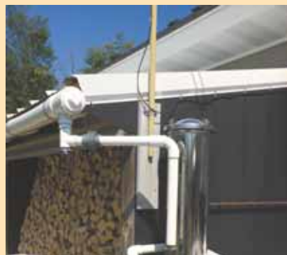
Smith cut notches into 4-in. pvc pipe and attached it to the eaves of his garage. Water flows off roof into a drop pipe that's plumbed to a pool filter, and then into tanks.
