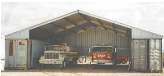
Fire station garage was made by setting a pair of 40-ft. shipping containers 32 ft. apart and installing a steel roof over them.
