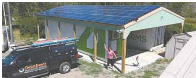
Kim Curren grows fresh, organic vegetables in refrigerated freight containers. They're housed in an open-sided pole barn, with a roof covered in solar panels.
