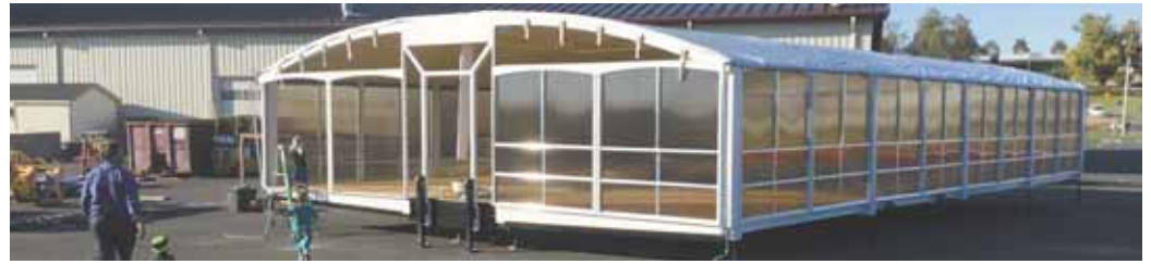
Portable wedding house measures 35 by 60 ft. and seats up to 400 people. It's built with light weight metal framing and polycarbonate windows.
