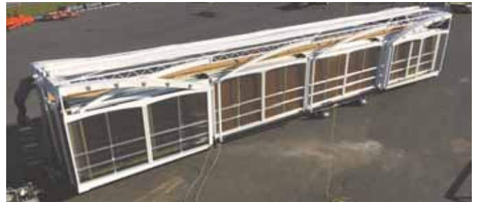
Building folds to a 9-ft. width for transport.
