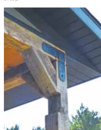
"Bilyeu fashioned forged iron straps and braces to attach and hold some of the posts and boards in place."
