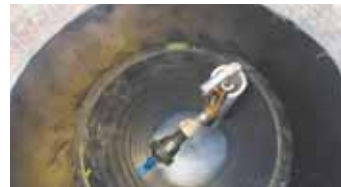
Scale model of remote valve and float control on water pipe at bottom of culvert.
