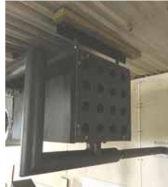
"Capture the Heat" unit uses engine exhaust to heat buildings. Exhaust enters box filled with baffles, then exits out the bottom and is piped outside.
