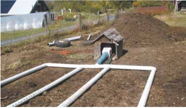
“Static pile” method of composting eliminates the need for stirring. Four 30-ft. lengths of 4-in. dia. pvc pipe are connected to a cross pipe “manifold” attached to a squirrel cage furnace fan.
