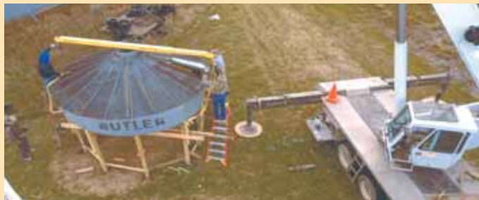
He bolted a series of 10-ft. stud walls onto silo all the way around. A deck below top of silo is accessed by a wooden stairway built inside silo.
