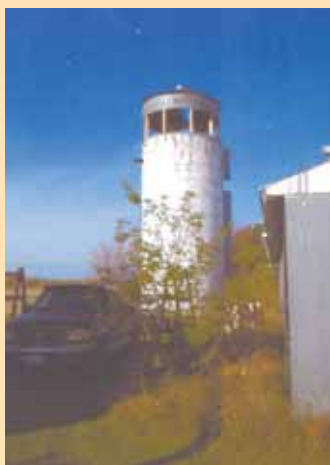
Peterson mounted the roof and upper ring off an old grain bin on top of his 28-ft. tall silo. A crane fitted with a horizontal steel beam was used to lift bin assembly onto silo.
