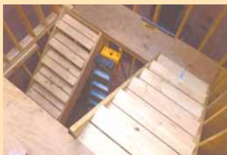
He bolted a series of 10-ft. stud walls onto silo all the way around. A deck below top of silo is accessed by a wooden stairway built inside silo.
