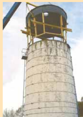
Peterson mounted the roof and upper ring off an old grain bin on top of his 28-ft. tall silo. A crane fitted with a horizontal steel beam was used to lift bin assembly onto silo.
