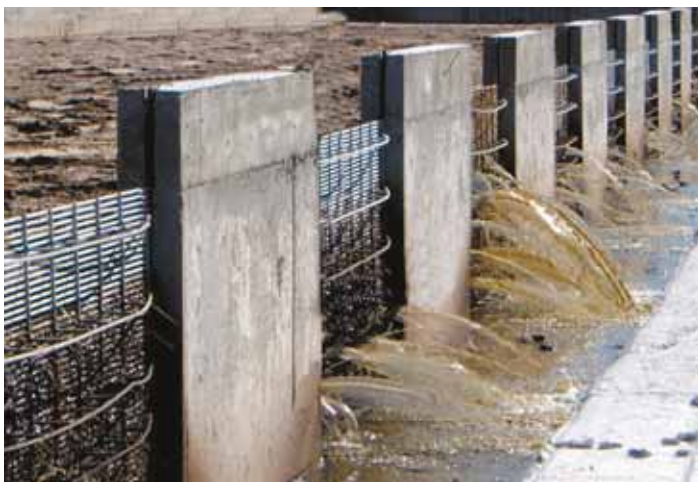
Steel hog flooring panels serve as “weep walls” that allow liquids to drain away from the stored manure.
