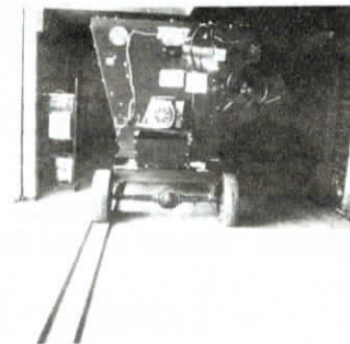
Track bolted onto floor guides mixer under silo chutes and overhead feed storage bin.
