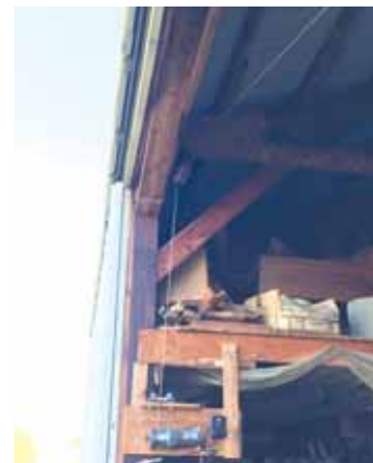
Wall-mounted 12-volt ATV winch does the lifting.
