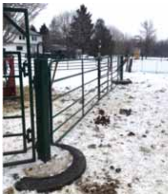
Temporary fence posts were made by setting wood posts in tires filled with concrete.
