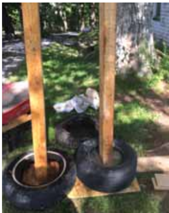
Temporary fence posts were made by setting wood posts in tires filled with concrete.
