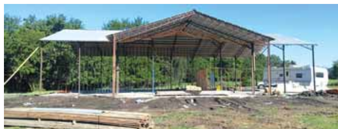
David Foster tears down old livestock buildings and sells the components. Photo shows a house under construction.
