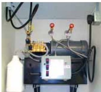
Built-in cleaning system's main unit is centrally located in an out-of-the-way spot, with remote "quick-connect" plates installed on walls anywhere you want.
