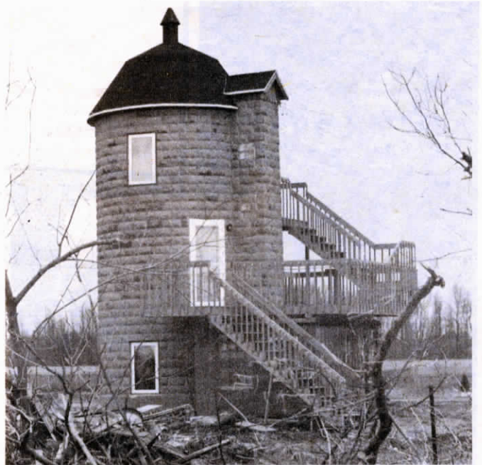
An old concrete block silo was transformed into this three-bedroom facility for overnight guests at a Dominican retreat center for spiritual growth near Denmark, Wis.
