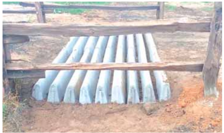
Reusable plastic forms make rounded beams with 4 1/2-in. gaps between them, which narrow to 2 in. wide at the base to prevent hooves from getting trapped.
