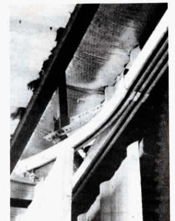
Front carrier on each door rides on inside track, the rear on outside track. Note space for air to enter barn on each side above the track.
