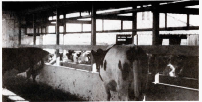
Note posts set inside feed bunk to minimize breakage, injury.
