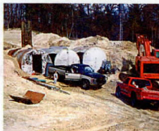
Fuel tank house is set into a hill overlooking 300 acres of crops.
