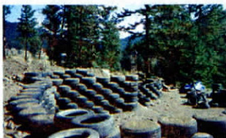
Tires are stacked flat and rammed full of dirt.
