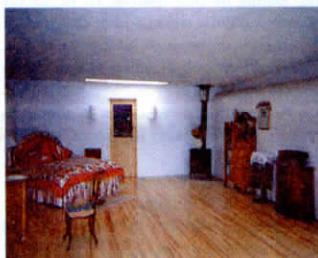
Interior walls of tire house are finished with adobe.
