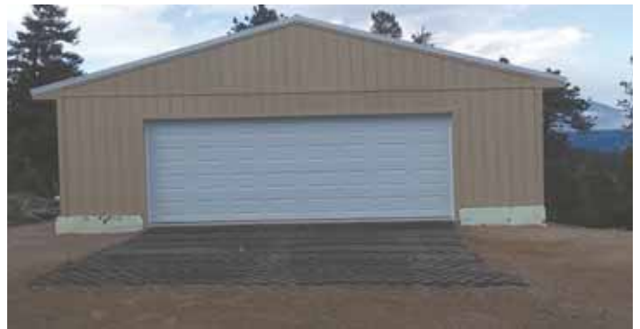
Jaime Stuever used lengths of bulldozer rubber track tread to make this 16-ft. wide, 27-ft. deep "tire tread" apron in front of his new workshop. "It saved thousands of dollars in concrete work," he says.
