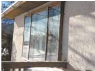
Lacey built "exterior" storm windows around his existing windows to cut winter heat bills.
