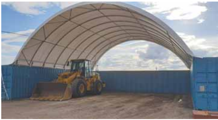
Canopy kit ties a pair of shipping containers together to create a low-cost, portable storage facility.
