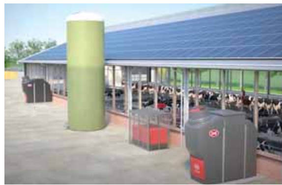
Photo shows N-Capture ventilators (far left and right), acid storage (small unit), and fertilizer silo for storing ammonium nitrate or sulfur nitrate.
