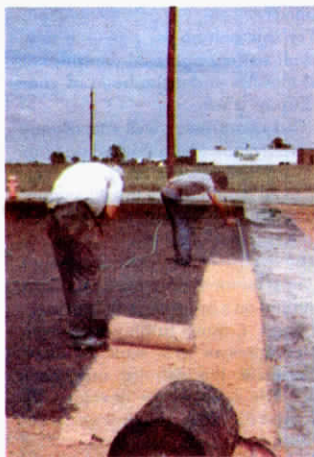
Individual mats made of chopped straw are 2 ft. wide, 25 ft. long. They're laced with a grass seed mixture and held together with a special bonding agent.
