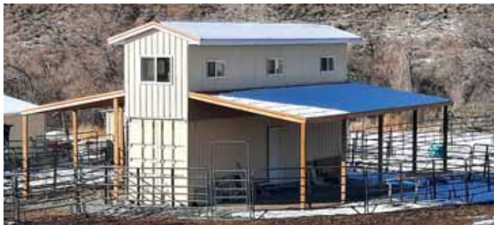
Chris Kornkven's 2-story horse barn is actually a used shipping container with a metal storage room built over the top, and 14-ft. wide lean-tos on both sides.
