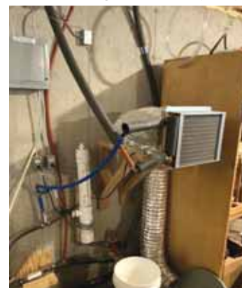
Water enters and exits the firewood-holding grate through separate outlets at the front. Heated water is pumped down through PEX pipe to a 12-in. sq. “water to air” heat exchanger in basement (below).
