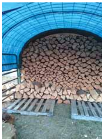
Dennis Althoff made these temporary firewood sheds by using 10-ft. corral panel for the walls, then installing stockade panels over them and adding tarps.
