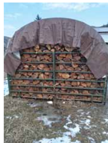
Dennis Althoff made these temporary firewood sheds by using 10-ft. corral panel for the walls, then installing stockade panels over them and adding tarps.
