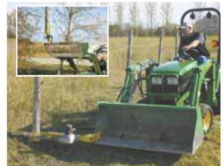
Hydraulic-powered cutter attaches to loader bucket.
