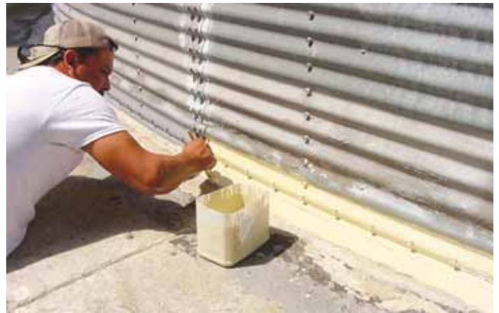
PermaFlex can be used to seal the base of grain bins, grain bin roofs, chicken coops and livestock floors to create a heavy-duty waterproof surface.
