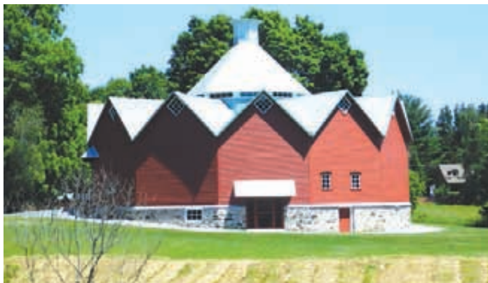
This 1881 wood and metal barn has 12 sides and a basement for free-roaming livestock with hay lofts along the outer walls.
