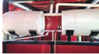
Water is collected from a v-shaped roof system and stored in barrels.
