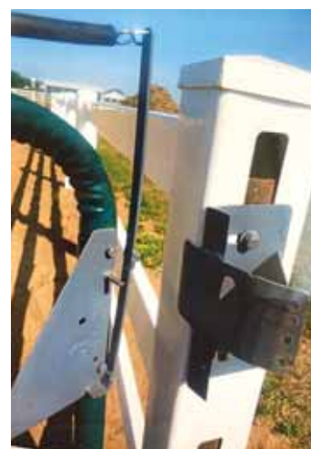
Gate hinge allows a horse rider to open or close a gate without dismounting.
