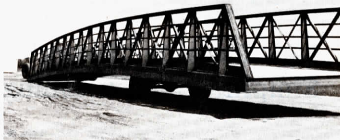
Pohlig says larger bridges are easily moved with a simple two-wheeled “dolly” as shown with this bridge awaiting delivery at Continental's factory.
