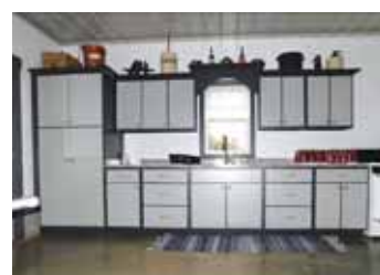
Miller has built many cabinets and one-piece window trims and other trims for many bathrooms, all out of HDPE plastic.
