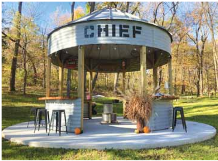
Jamie Dougherty converted an old 18-ft. bin to a gazebo complete with cedar slab countertops.
