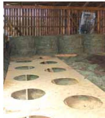
Bales rest on an elevated wood platform with holes in it. Hot air from the roof blows up through the bales.
