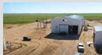
The Varcor manure processor is housed in this building. Ammonia vapors are siphoned off and used as a heat source for the evaporation process.
