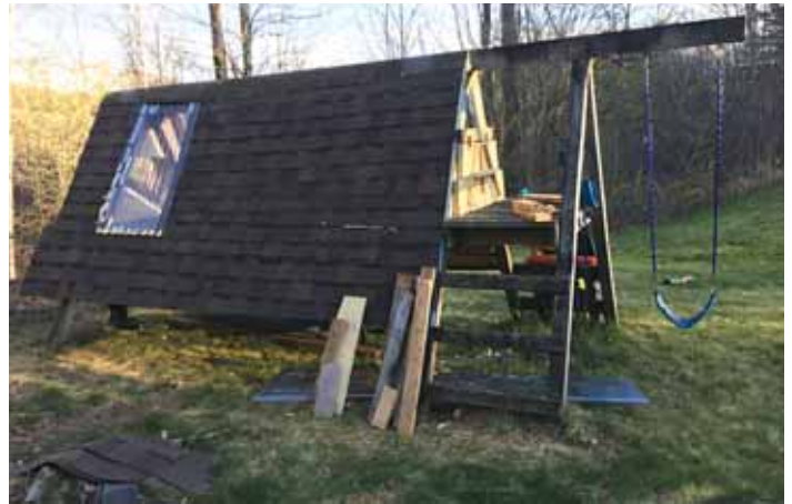
The chicken coop was built using an existing swingset. It has a corrugated plastic "window" and removable door for feeding and clean-out at one end.
