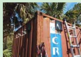
**The 360 Tunnel system uses an intake port and exhaust port on shipping containers to move air, even in low wind.**
