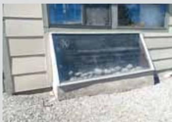
**Rick Bohl, Cedaredge, Colo.:** “I made a passive solar heat collector for my shop by using a section of salvaged sliding patio door. I cut air intakes into each end near the ground and cut a hole into my shop near the top corner of the collector. A small fan pulls air into the shop, at the same time drawing air into the solar collector through the air intakes. The fan came from a kitchen vent in an RV. Its speed is regulated by a light dimmer switch.
