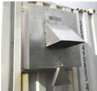
Air Cleaning Blowers work without filters. Air pressure spins particles off to the side.
