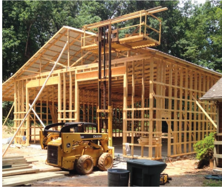
Industrial forklift mast attaches to skid loader arms and can be fitted with a 12-ft. long metal basket that slides onto the forks.
