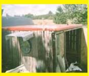
This little pallet lean-to sits on 4 by 4's and the walls and roof are framed with used pallets. The metal on the roof was left over from another project.
