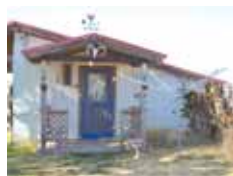
Main entrance after renovations.
