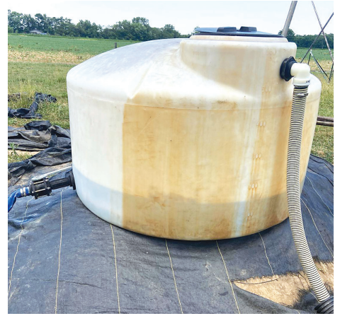
“The 550-gal. tank gives me 3 to 4 ft. of head pressure, sufficient for drip irrigation,” says Wood.
