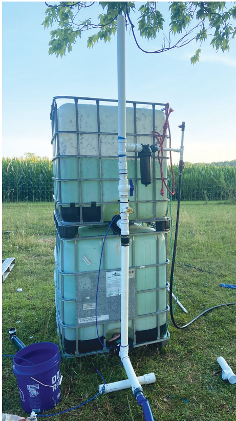
Wood placed two 270-gal. IBC totes, one on top of the other, on the highest point of his farm for a water tower.
